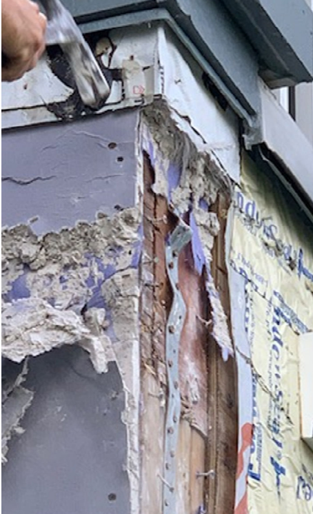
Figure 5. How do Straps handle shrinkage. They don't!
